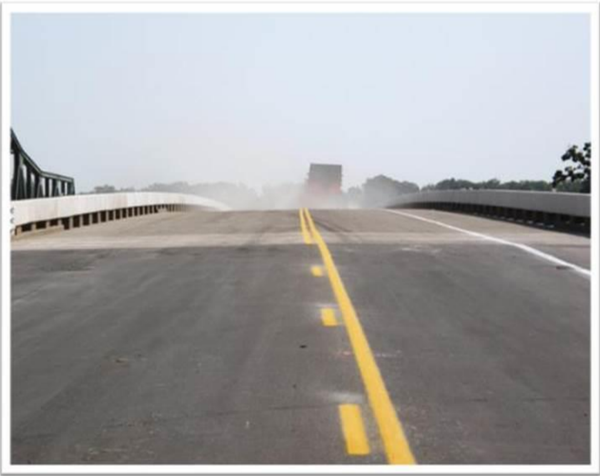
New K-47 bridge west of St. Paul prior to opening (old bridge at left)
